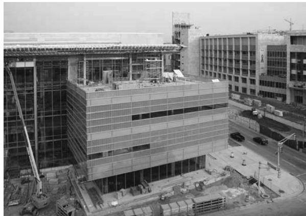
Campus Center construction, IUPUI
