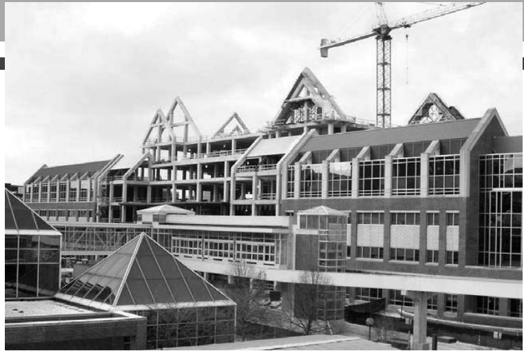
Research III construction, IUPUI
